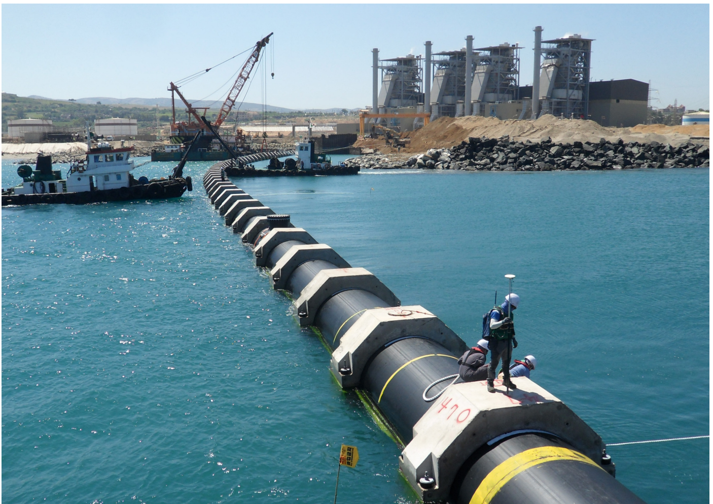
Beginning of submerging of OD2500 mm SDR26 pipe
