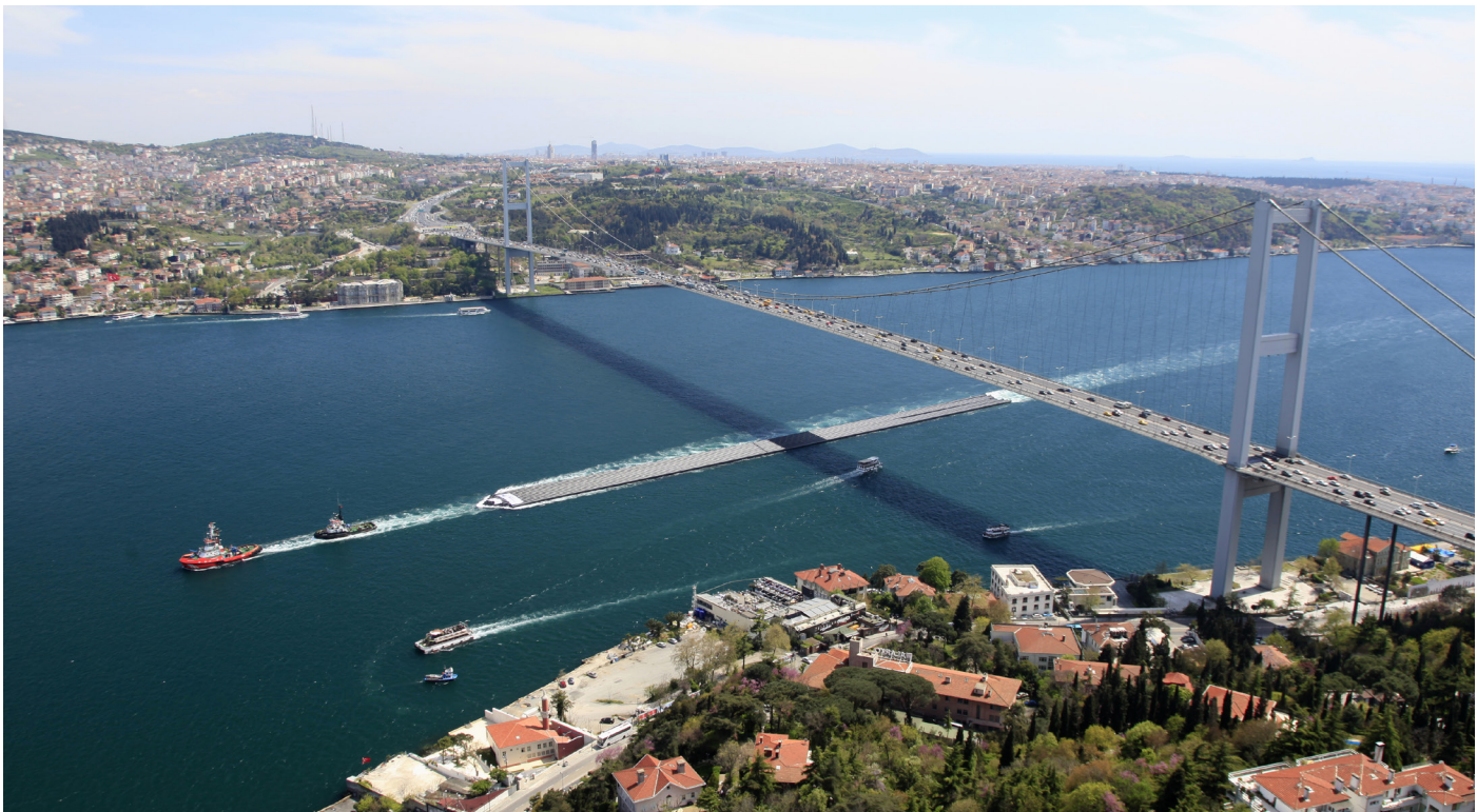
Pipe tow through the Bosphorus Channel
