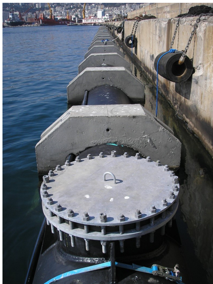
Completed saddle fitting with temporary blank flange
